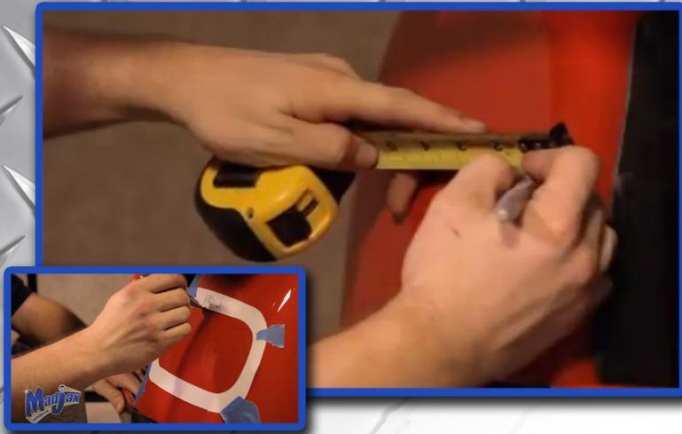
Using the measurements provided on your tail light template, measure and mark your template. Use a marking pen to trace the inside line. \*Flip template over to use on other side.
